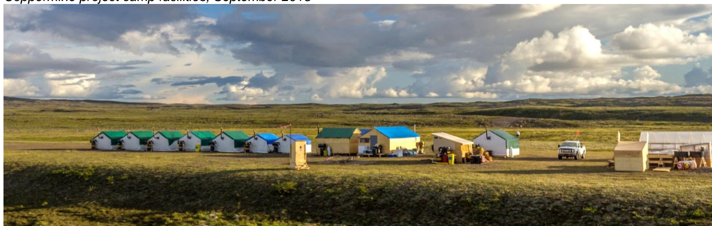
Coppermine project camp facilities, September 2015
